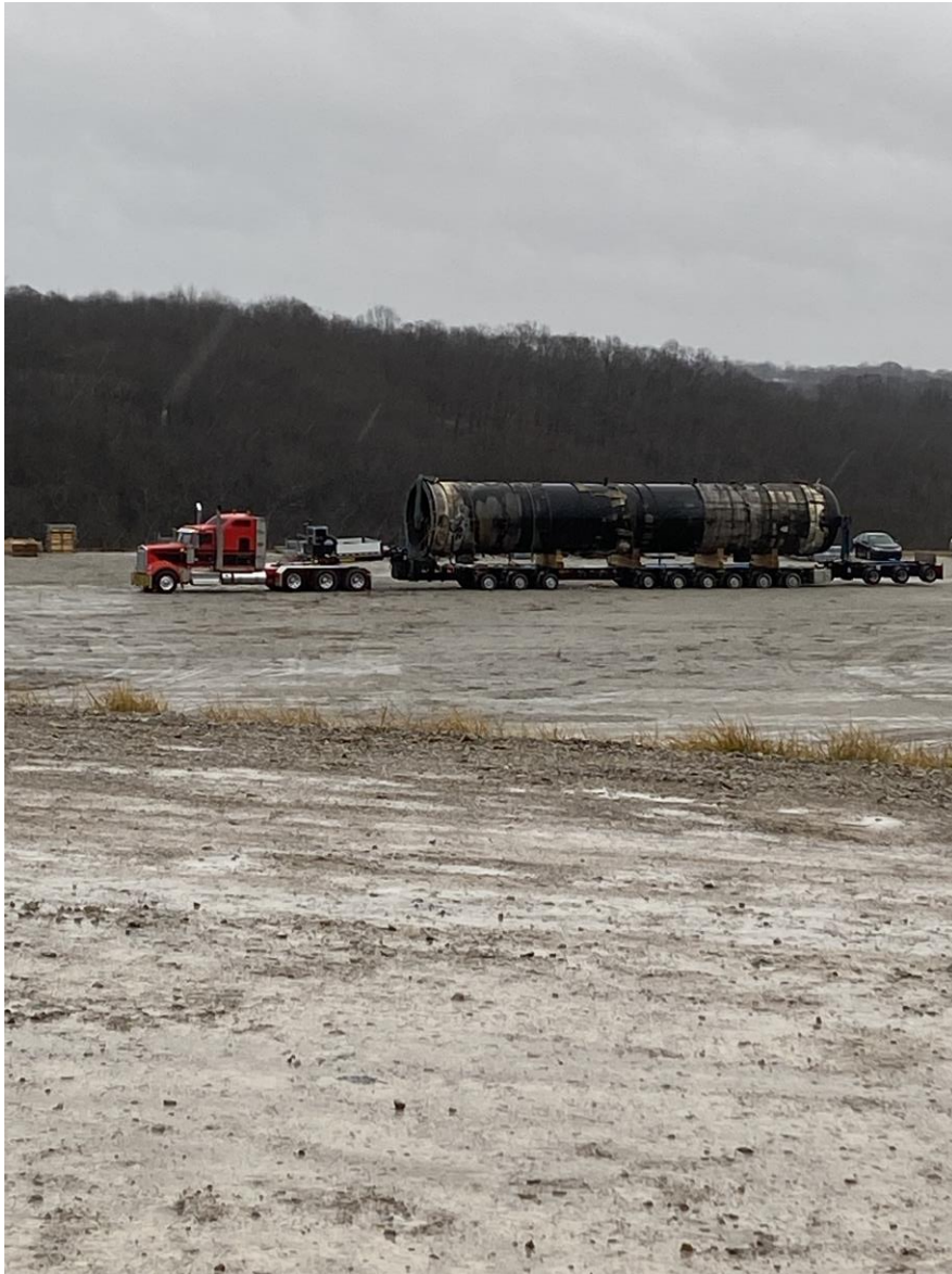
Photo 2 – amine system contact tower (had been in place on cement pad in photo #1 where person with gray shirt and brown pants in standing)
